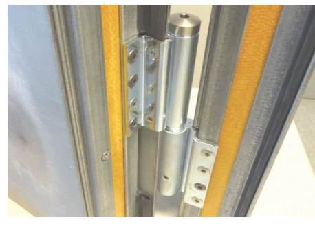
8) Hinge on fire-resistant profile
